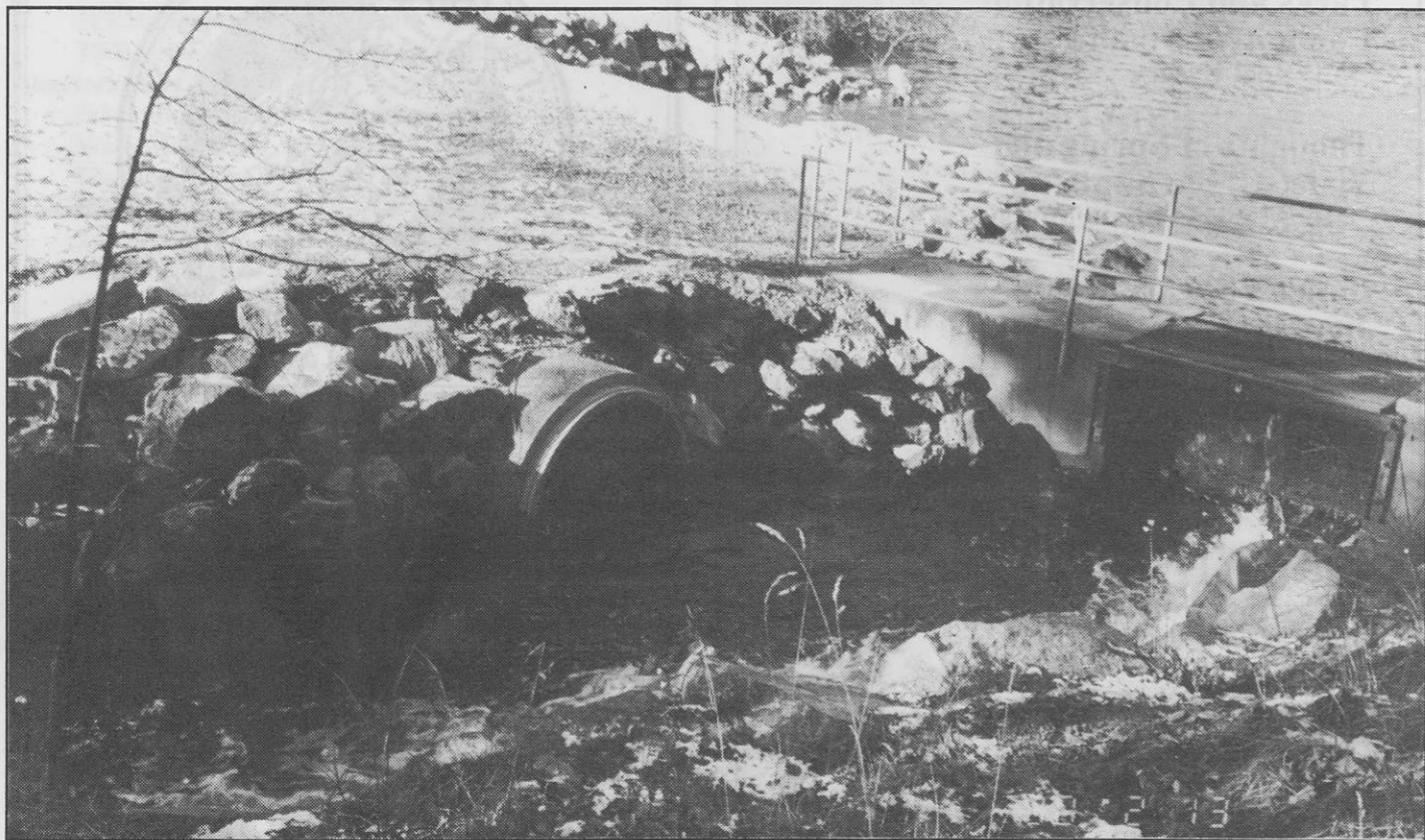
(Right, above) Weir at the outlet of Beaver Lake where it empties into Colquitz Creek. The concrete culvert (left) is a fishway which gives spawning Cutthroat Trout and their fry unrestricted access to the waterway.
